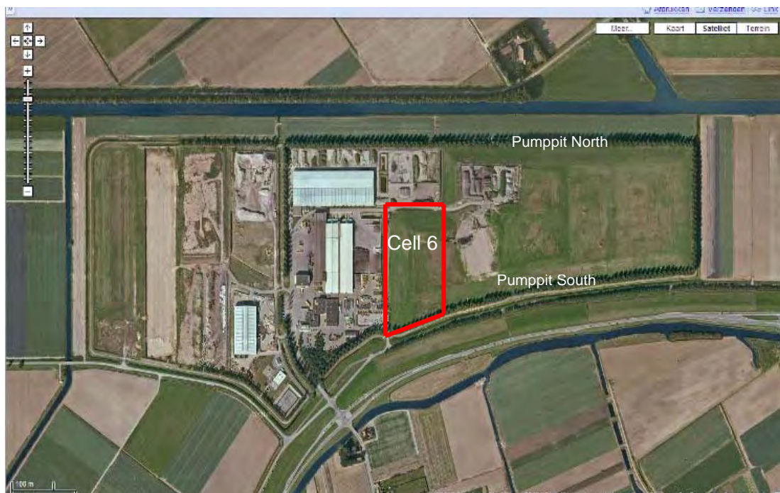
Figure 4.3 Selected waste cell 6 for demonstration project and two leachate collection pump pits
