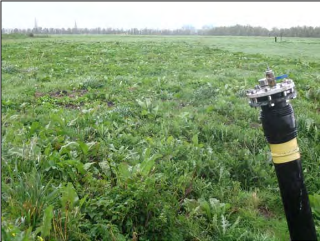
Plateau of cell 6 and gas well
