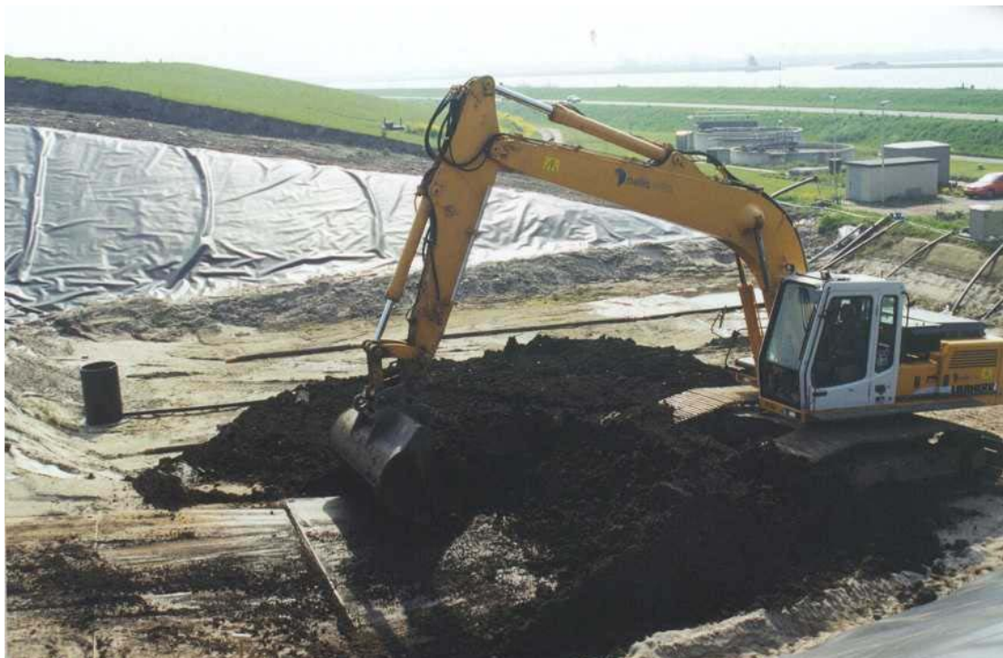
Figure 5 Overall view of the building of the pilot project at Nauernasche Polder. A bottom liner can be seen at the side of the cell. The waste was placed in layers with an excavator. Steel planks were used to safeguard the mobility of the crane.
